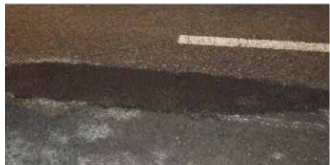
Images of cold lay materials, before and after, courtesy of TfL
