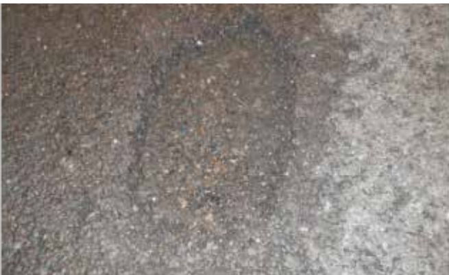
Images of cold lay material, before and after, courtesy of TfL
